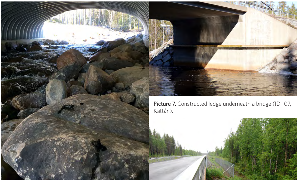
Picture 6. A new dry bank created underneath a bridge. Otter spraints can be seen in the picture (ID 309).
