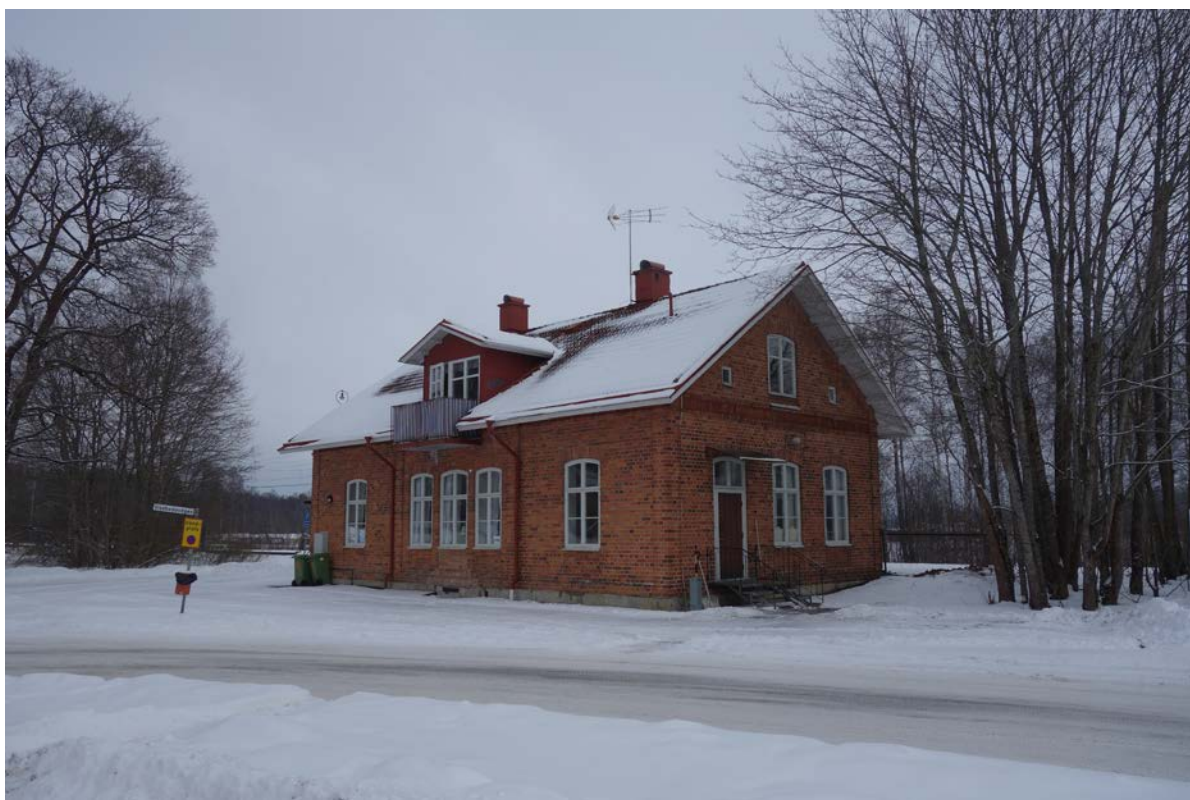
Figur 4.13 Stationshus i Asbro
