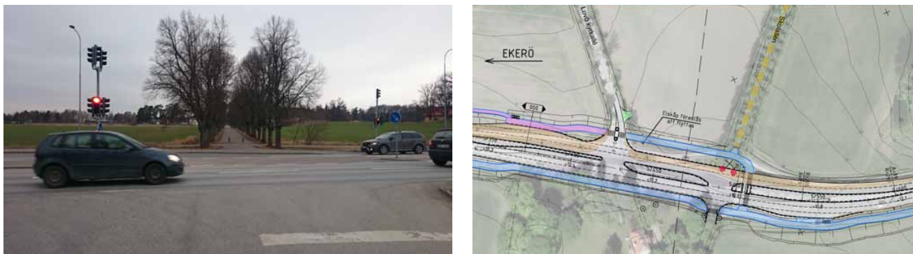
Fig. 4.6 a, b: Existing situation of intersection between Ekerö Road and Lovö Kyrkallé and planned design of the intersection of Ekerö Road with Lovö Kyrkallé and Skolallén at Canton (© Michael Kloos / Swedish Transport Administration)
