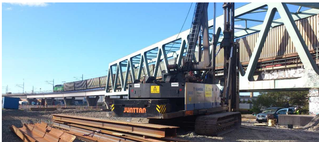
Figur 12 Pålmaskin, P1. Maskintyp: Junttan Pile Driving Rig PM23(1).
