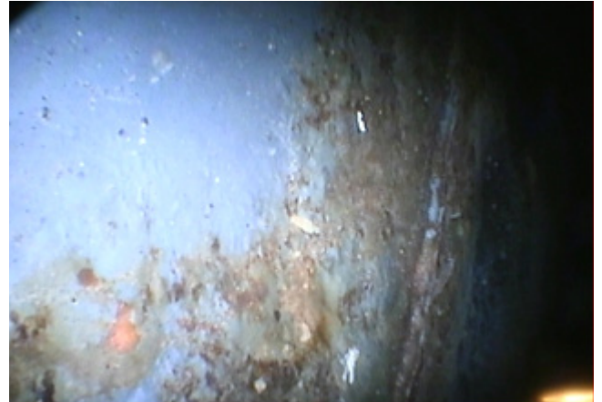
Figure 45. Frame beam left front inside.
