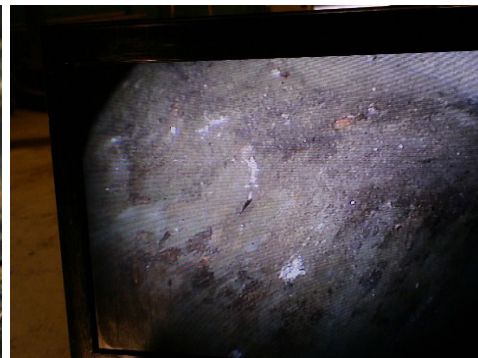
Figure 37. Frame beam left front inside.
