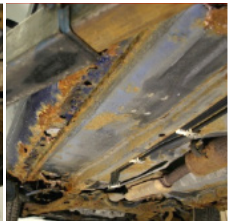
Figure 31. Left side beam outside.
