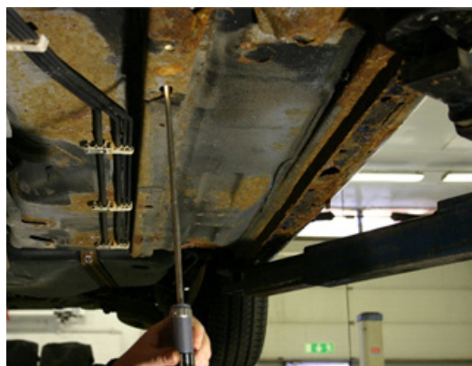
Figure 32. Camera entry point left side beam.
