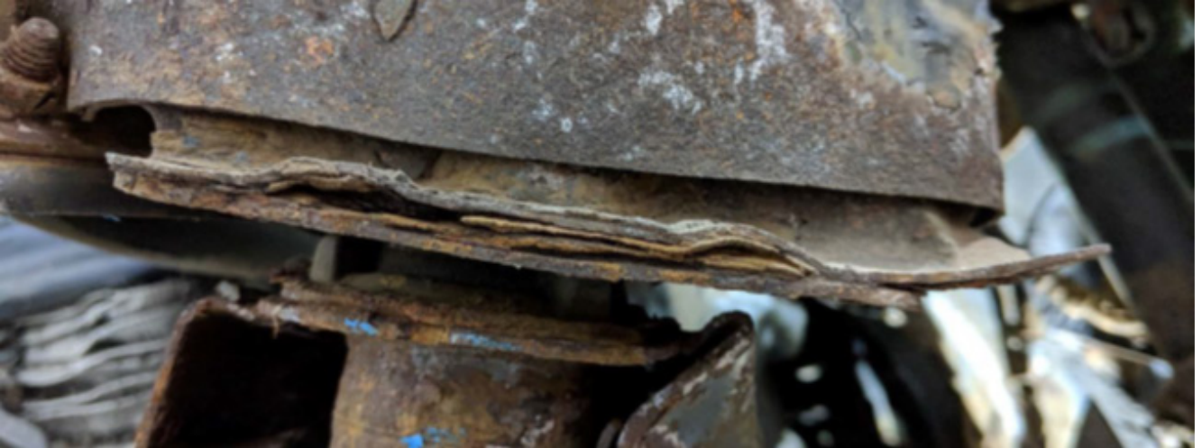
Figure 56. Frame beam underside
