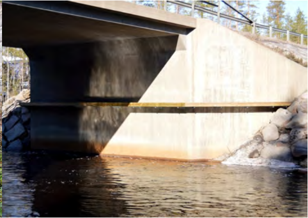
Figure 3. A constructed ledge at Kattån river (ID 107).
