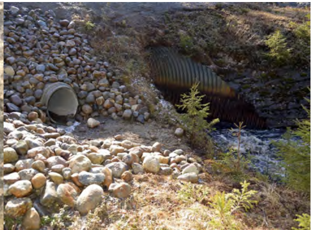
Figure 5. A dry culvert with complementary structures, Röjavattsbäcken Creek (ID 196).
