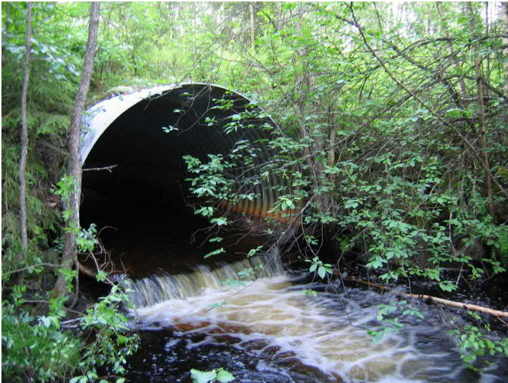
Picture 2a. Object 44 before, culvert with a fall at the outlet.
