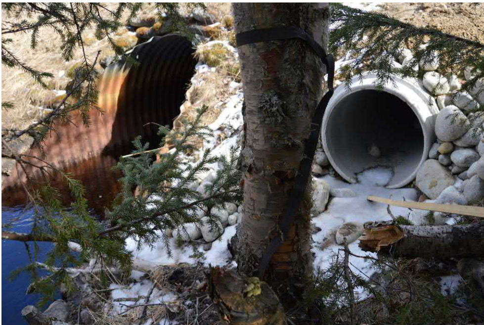
Picture 3b. Otter mitigation, a dry culvert for otters to go through, object 197.
