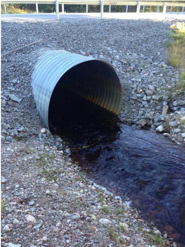
Picture 4b. Object 59, after, a culvert which is lowered and increased in dimension. Material is put in to the culvert to let the riverbed continue under the road
