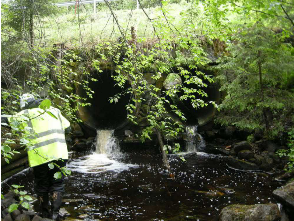
Picture 1a. Object 191 before, culverts with falls in the outlet.
