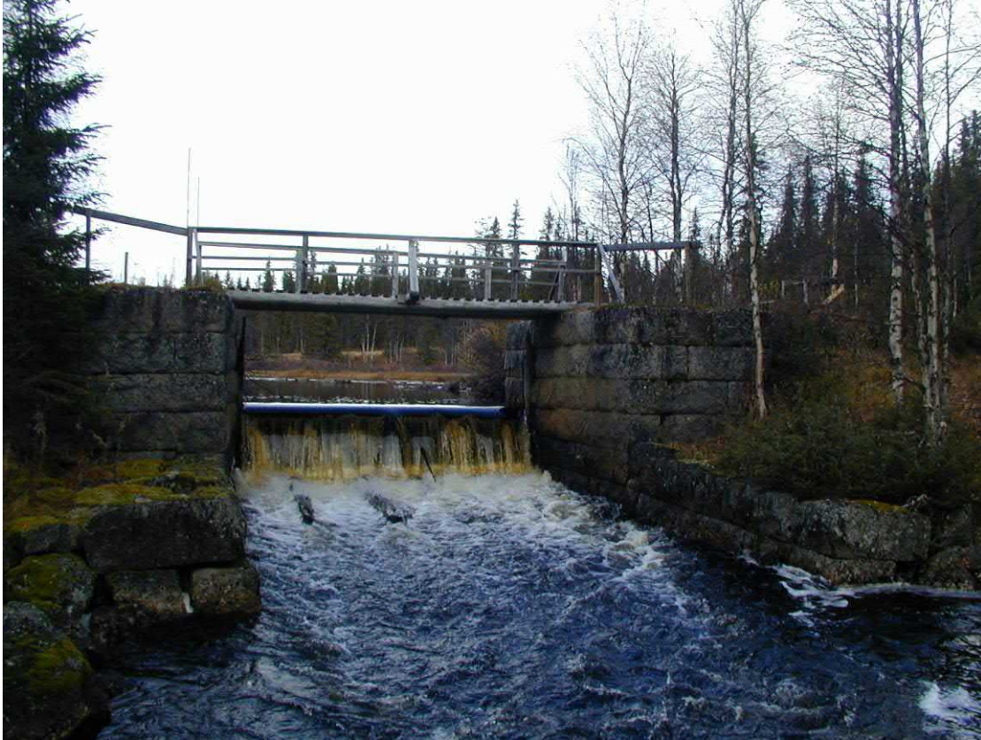
Picture 5a. Object 173, before, a dam that is a migratory barrier for fish
