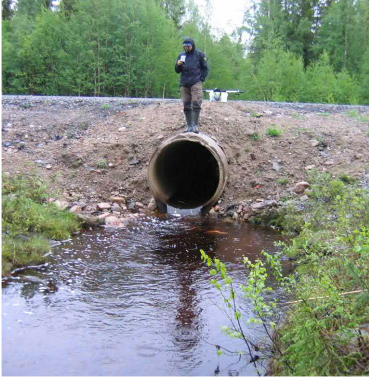
Picture 4a. Object 59, before, a culvert with a fall at the outlet
