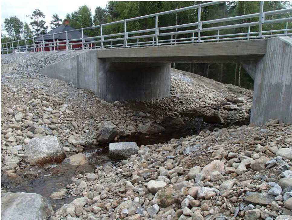
Picture 1b. Object 191 after, bridge with a natural riverbed.
