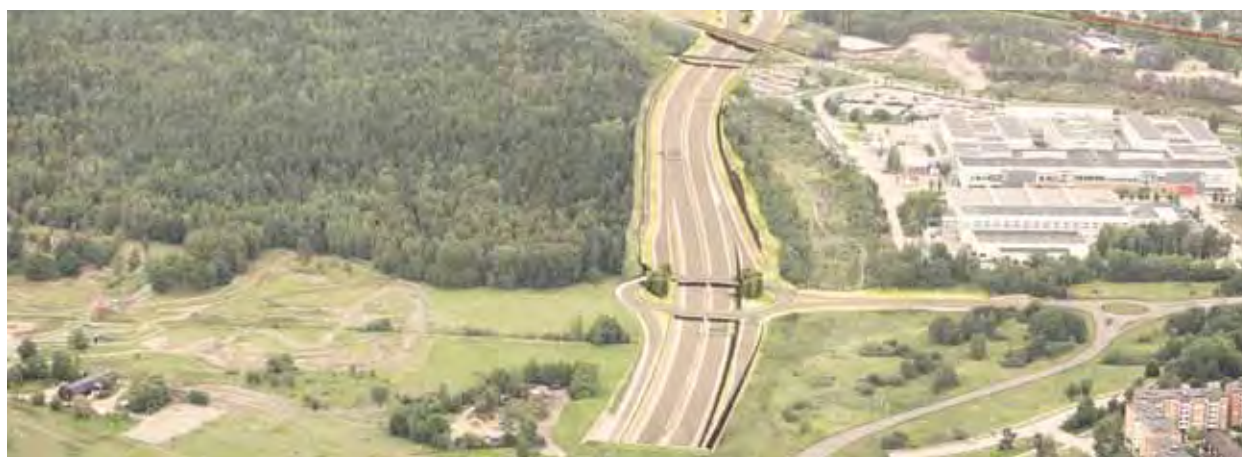
The Stockholm bypass runs in a deep trench north of Akalla. Thereafter it continues northwards under the Akalla interchange towards Häggvik. The Akalla interchange links to the Hanstaleden thoroughfare.
