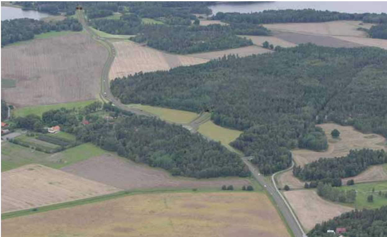
Interchanges by Edeby and Tillflykten on the Lovö island seen from the north.
