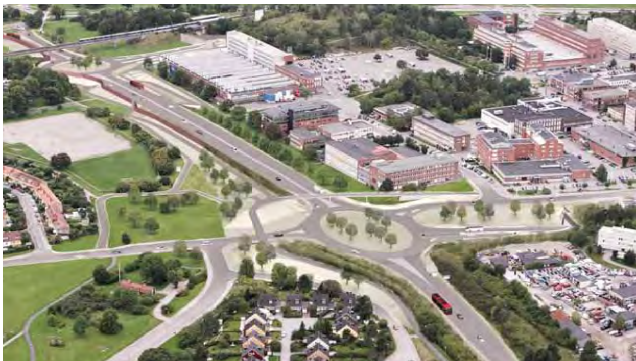
Vinsta interchange seen from a new interchange on Skattegårdsvägen towards Johannelund and Berslagsplan.
